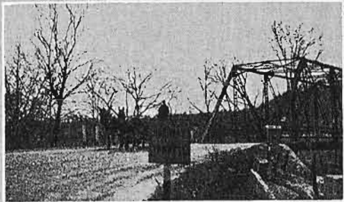
OLD SUGAR CREEK BRIDGE, NORTH OF BELLA VISTA. NARROW ROADWAY AND SHARP CURVE.
