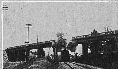
COTTON BELT OVERPASS AT KINGSLAND ON ROUTE 79. 342' CONCRETE AND STEEL STRUCTURE.
